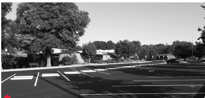
Repavement of parking lot at Barretts Elementary
