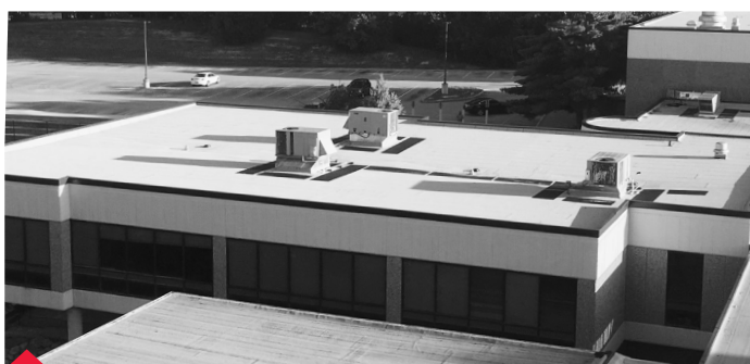
Central High roof replacement
