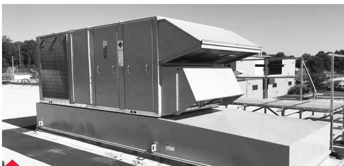
Central High HVAC replacement
